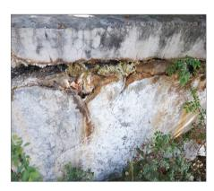
reinforcing bar is broken, the steel's passive layer will break down and active corrosion of the steel will start. There are two mechanisms, however, that will damage the passive layer on the steel reinforcement, even if the concrete cover is not damaged: chloride ions and carbonation. This makes the steel vulnerable to corrosion.
