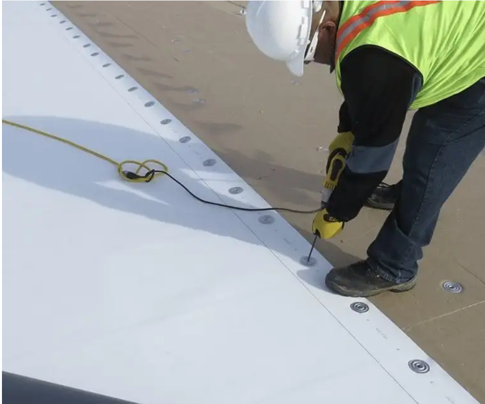
ANCHORING OF MEMBRANES
