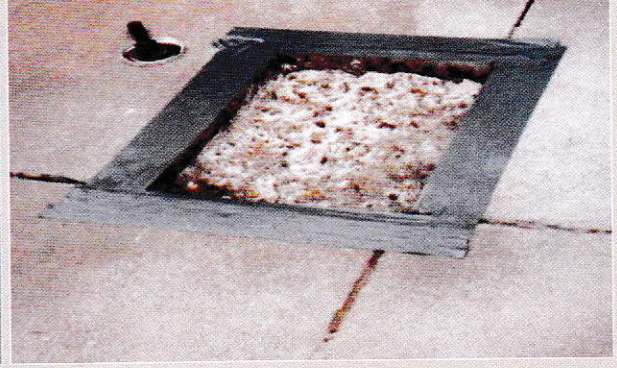
Application: Vacuum Cleaned Surface Ready for Shali Patch 10/20 Application
