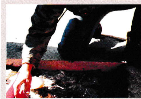
Application: Priming the Surface with Shali Prime PUM
