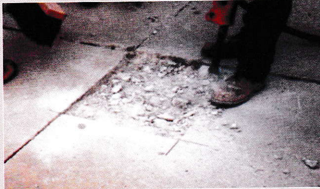
Application: Surface Preparation-Saw Cutting & Chiselling to Achieve a Rectangular Shape
