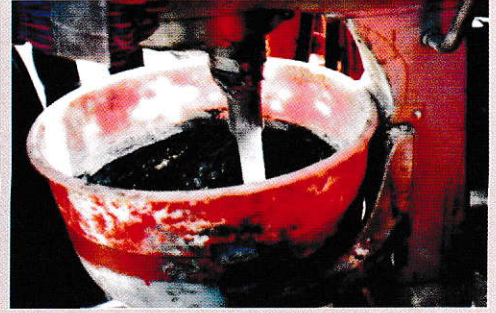
Application: Homogeneous Mixing of 3C of Shali Patch EC 10/20 with Electric Stirrer
